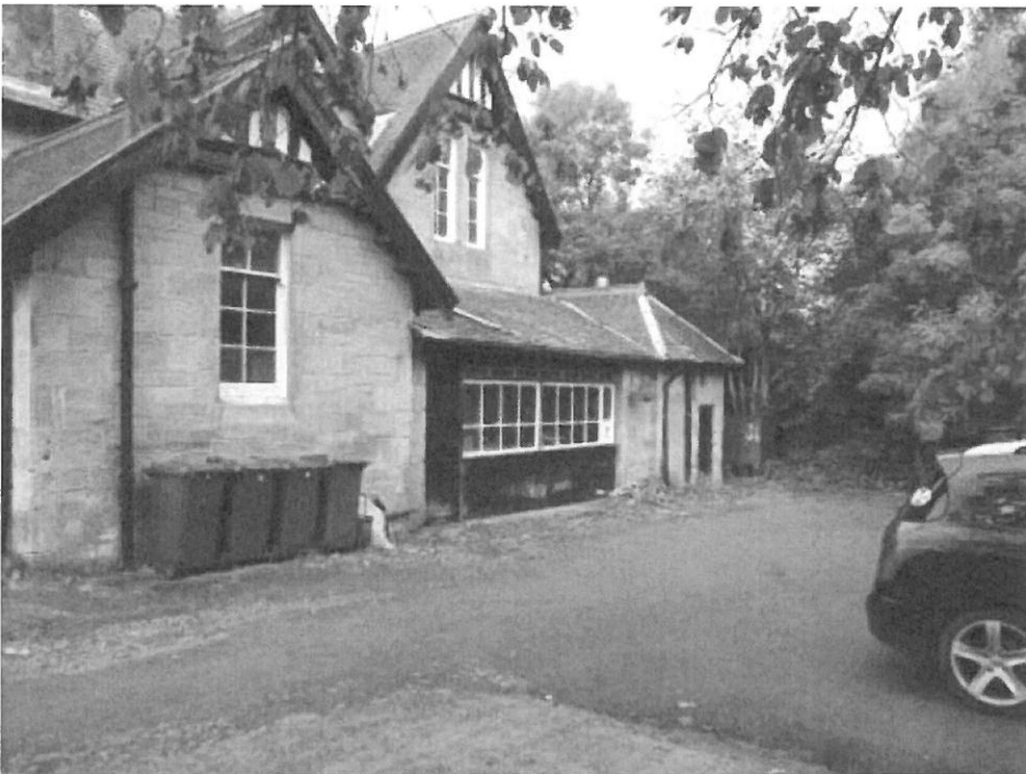
Photographs of 36 Peace Avenue, Quarriers Village
