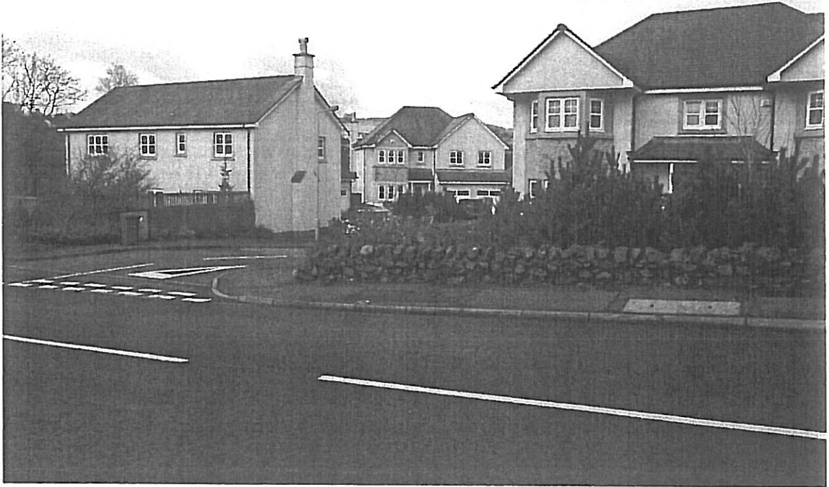
Adjacent development on the site of the former Pacemuir Mill.
