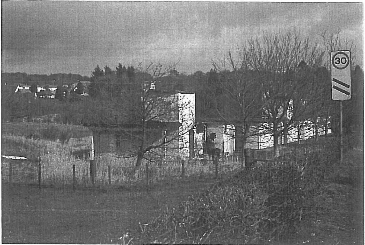
View of existing building from western approach to Kilmacolm (B786)
