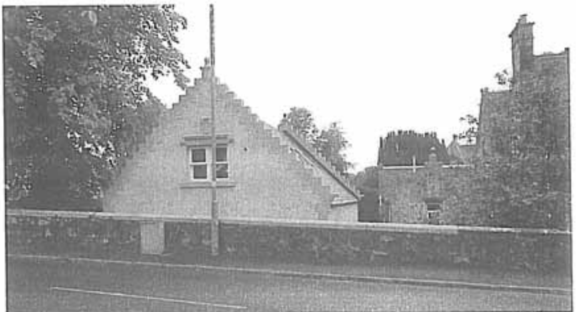
Photo 8 - Proximity of Garage to Torr Road in Conservation Area looking North
