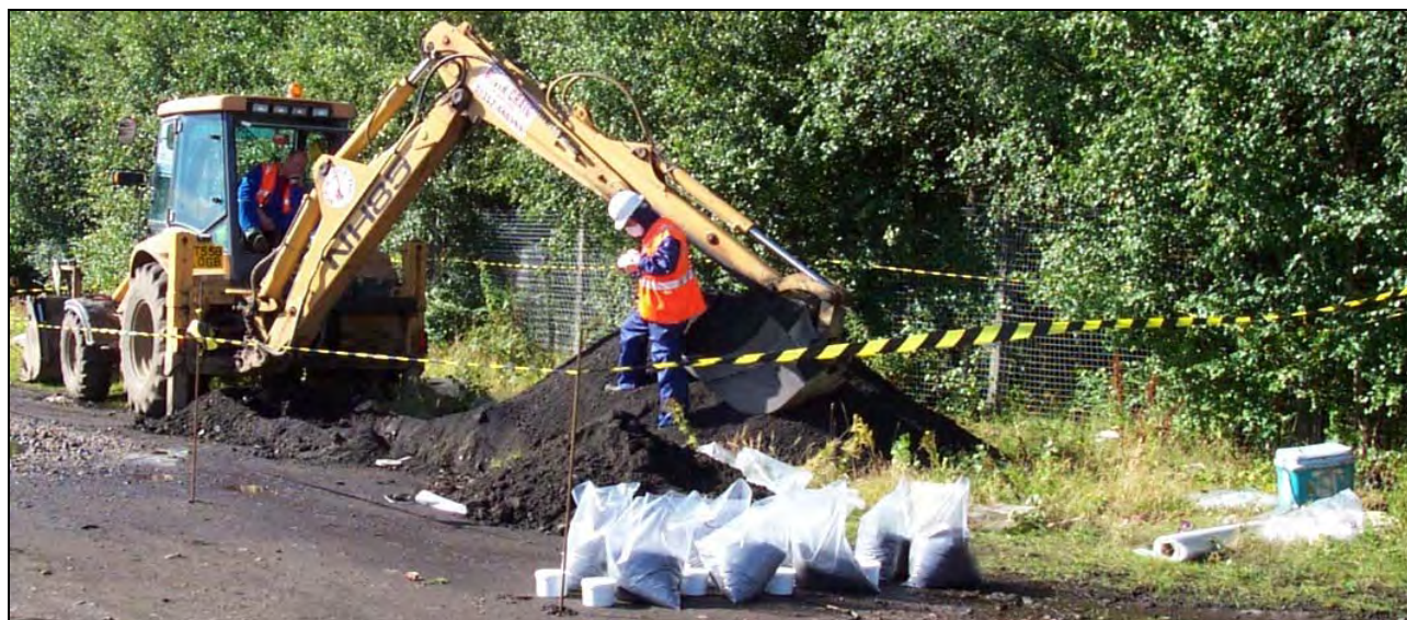
Trial Pit Excavations and Sampling
