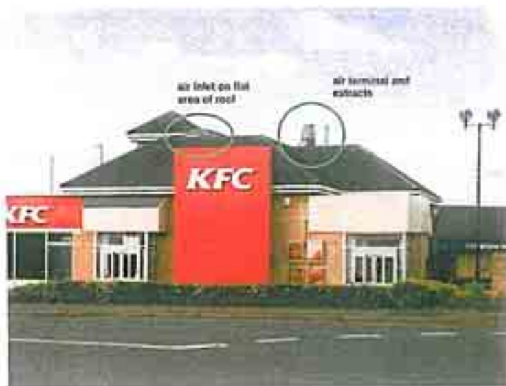
Fig 16: Example of cafe where air inlet and air terminal are exposed above roof. Note that although a flat roof has been installed to help conceal these elements, they are still visible.
