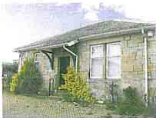
Fig 6: Photos of existing building
