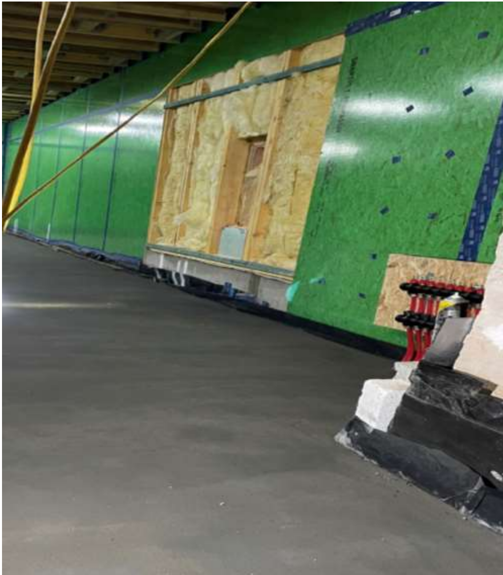
• INSULATION BEHIND SMART PLY
