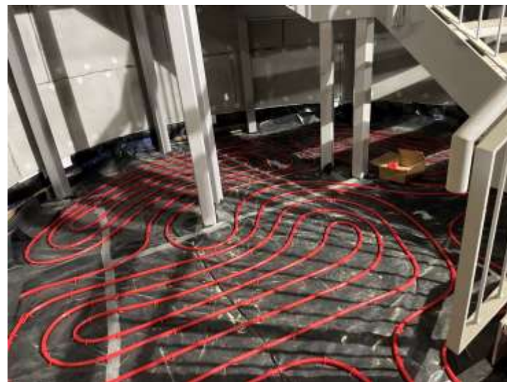
INSULATED UPPER FLOOR AND STAIR UFH
